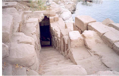
Photograph 2. The nilometer on Elephantine Island, Aswan, consists of stairs and staff gauges.
