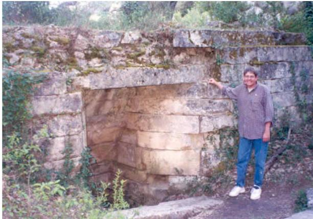
*Photograph 3. The intake for the penstock at Jean de Mare Mill.*
