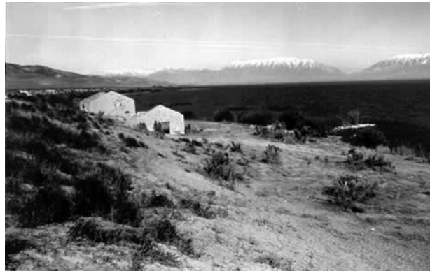
Photograph 1. The empty concrete shells of the pumping plant and engine house are still standing on the Utah Lake shoreline. Circa 1984.
