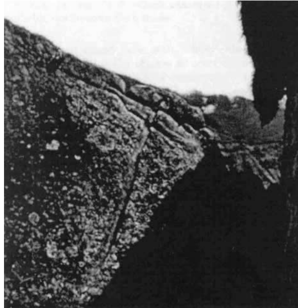
Figure 9. Drip Line Cut into Stone behind Southern Wayrona Near the Sacred Rock. Originally, Thatched Roof Extended Out to Drip Line.
