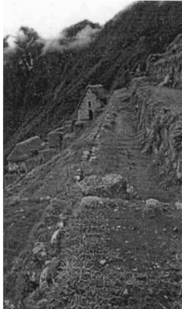
Figure 7. Canal with Qolqas (Storehouses) and Terraces in Agricultural Sector. Water Supply Canal and Agricultural Terraces Were Found in Good Condition by Bingham in 1911, Attesting to Excellent Engineering of Ancient Incas.
