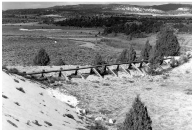
Photograph 4. All that remains of the third effort at putting a dam at Hatchtown is the spillway. In the background is Flake Meadow. Circa 1984.
