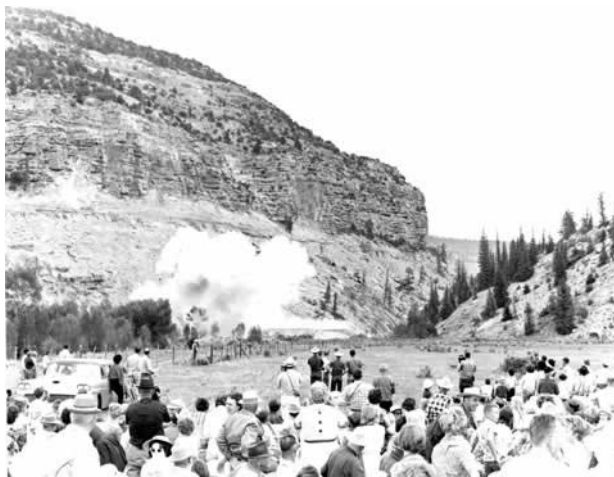
Photograph 4. Startled crowd views blast at the Joes Valley Dam groundbreaking ceremony(1963).
