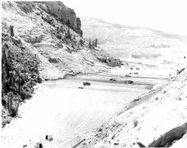
Photograph 7. Work progressing on the earthfill at Joes Valley Dam (1965).
