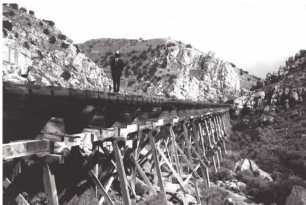
Photograph 4. An impressive flume was built down Goshen Canyon, sections of which were supported on a wooden trestle. Circa 1910.
