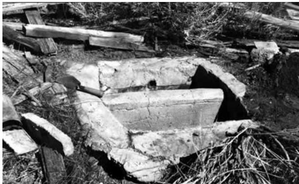
Photograph 10. Before water entered the cistern it was filtered in a small concrete box which contained sand and charcoal. Circa 1984.
