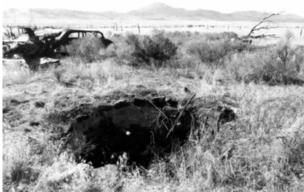
Photograph 9. Drinking water for Elberta residences was provided from cisterns located near individual homes. Circa 1984.
