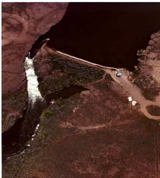
Photograph 3. Mona Dam and Reservoir as seen looking east from the air. Mona Reservoir provided water storage for the Elberta project. The dam is one of the oldest in the state of Utah. During the high snowmelt of 1983, it came close to overtopping. Sandbags (the long white line) had to be brought in to raise the freeboard. Circa 1983.
