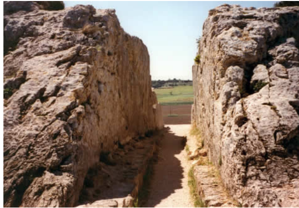
Photo 2. The cut for the channel that delivered water to the mill at Barbegal.
